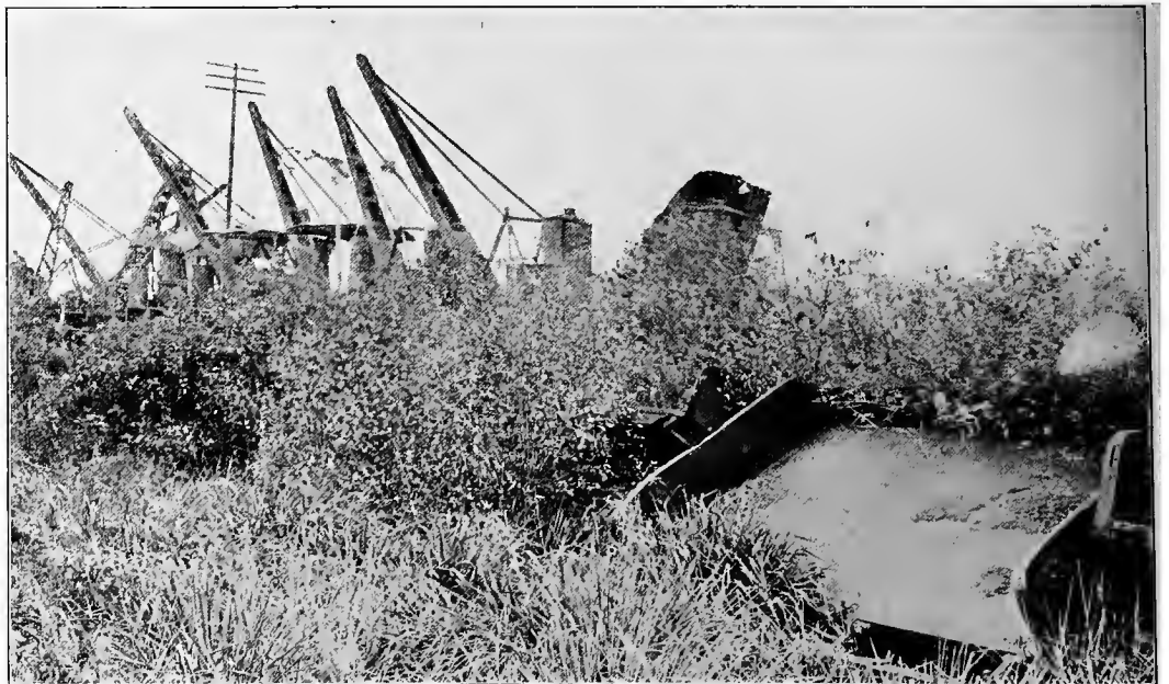
MACHINERY SEEMINGLY AS HOPELESS AS THIS WAS RECOVERED AND SET TO WORK
